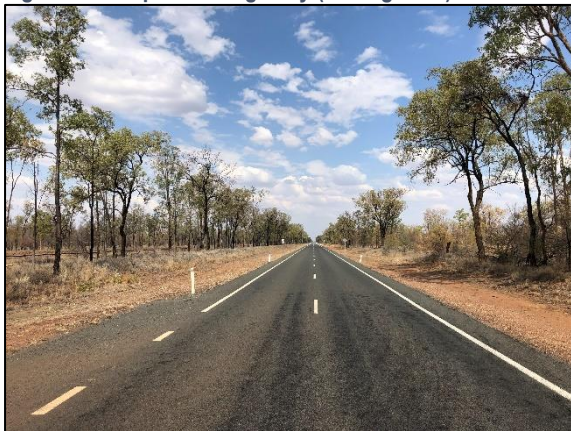
Figure 3.1: Capricorn Highway (Facing East)
