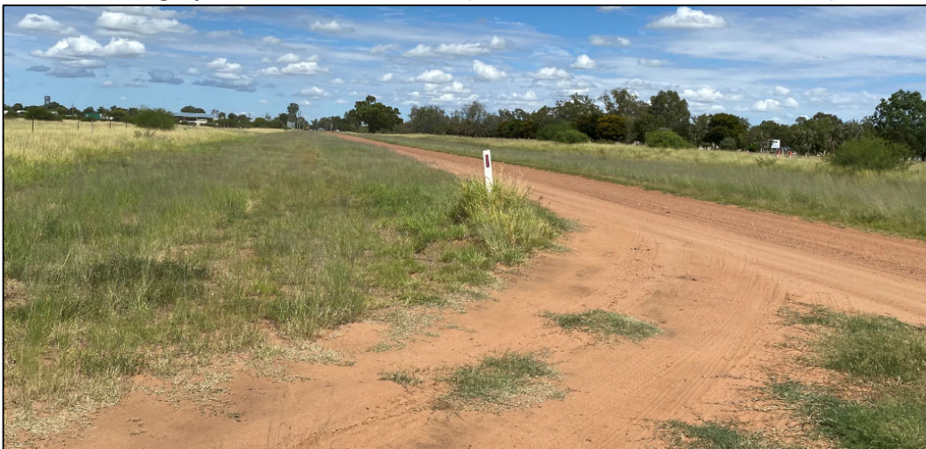
Photograph 2 – Lancewood Road (view west from Beefwood Road)
