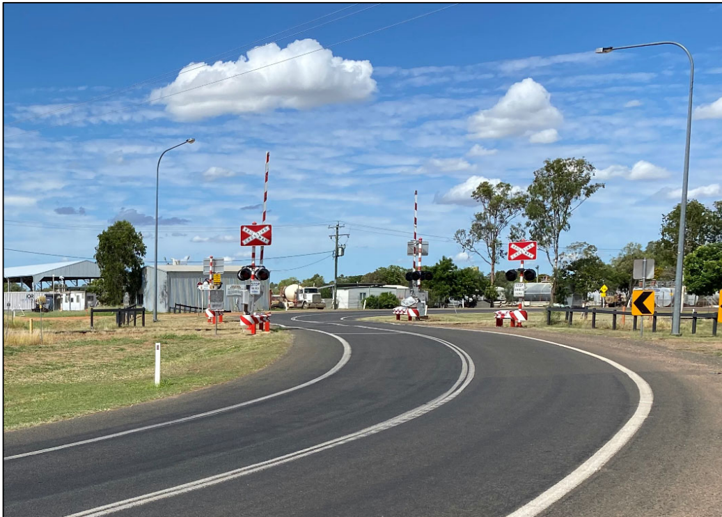
Photograph 13 –Railway Level Crossing
