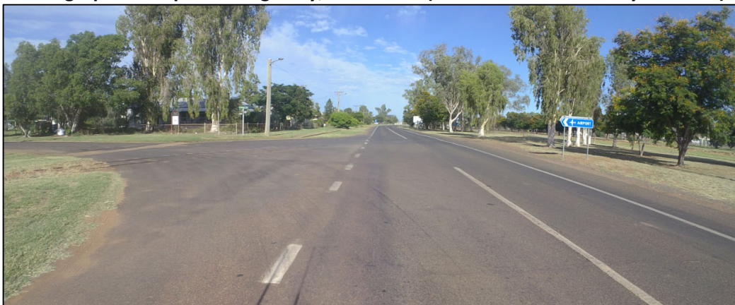
Photograph 7 – Capricorn Highway/Oak Street (at intersection with Myall Street)
