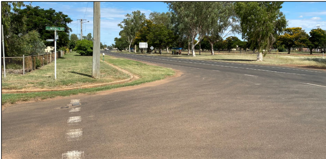
Photograph 11 –Oak Street and Myall Street, Sight Visibility (View West)
