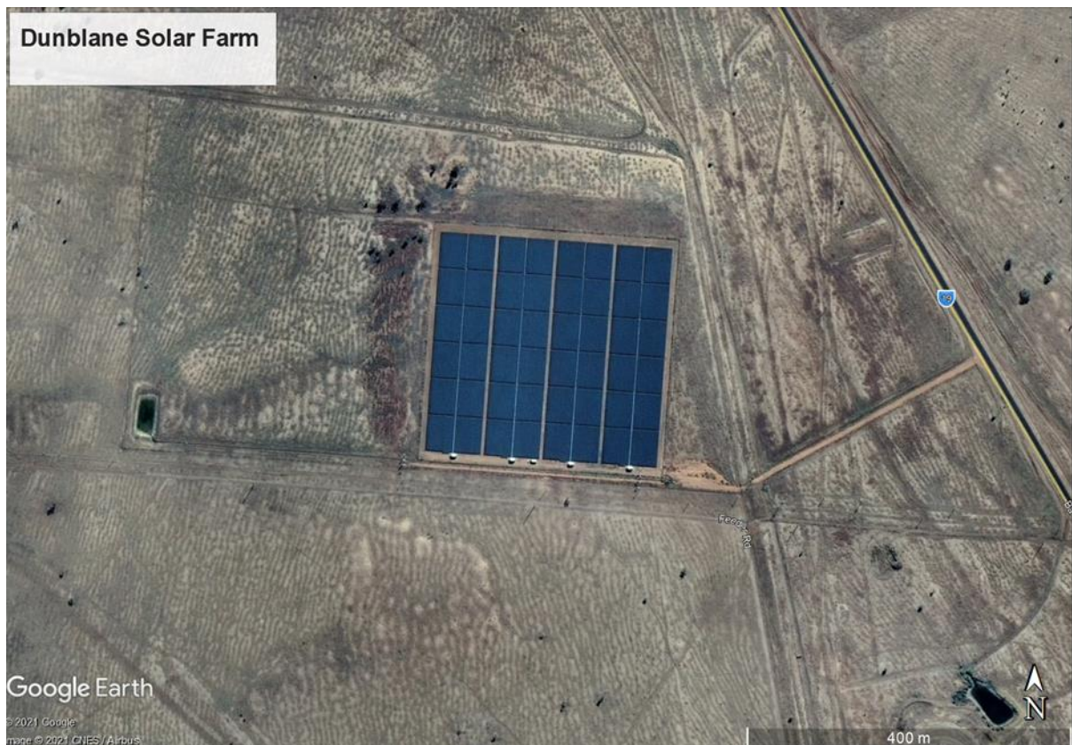
Figure 1: Dunblane Solar Farm
