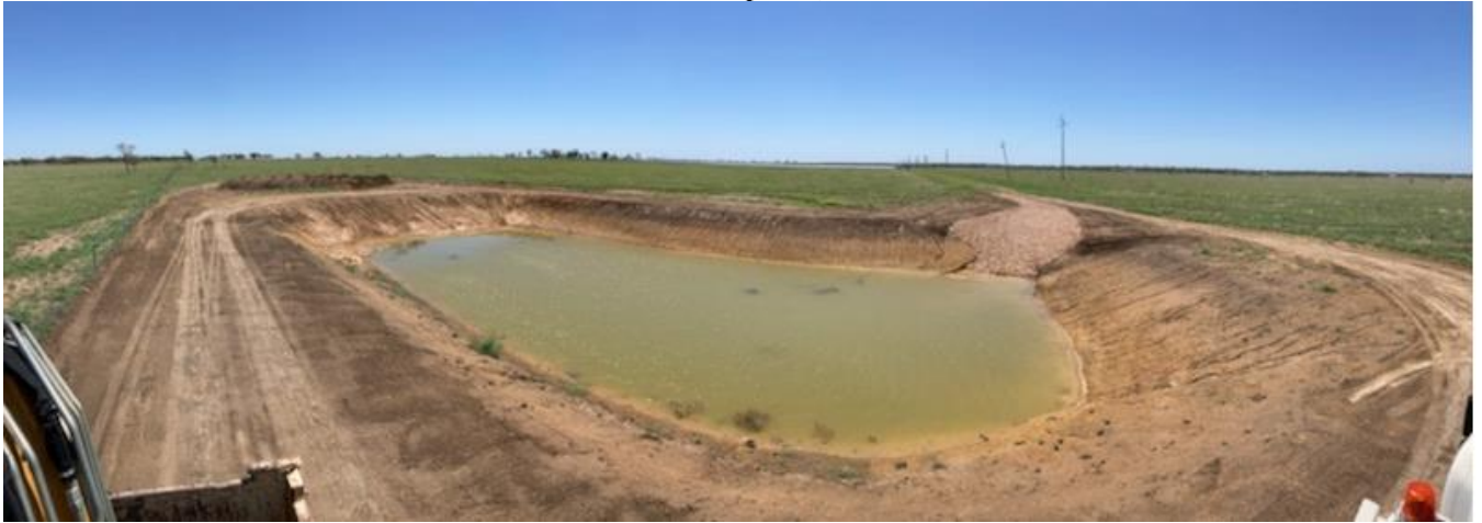
Figure 4: Landscape view of detention pond looking northeast showing ground level bywash on western side (left side of photo)
