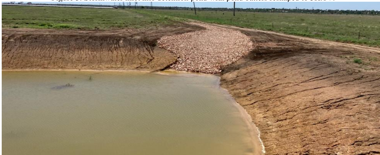
Figure 3: Stormwater inlet into detention pond with pond batters reshaped to 3H:1V.
