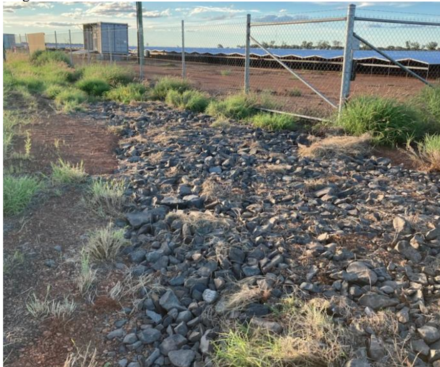
Figure 1: Eastern end of stormwater drain with additional rock material
