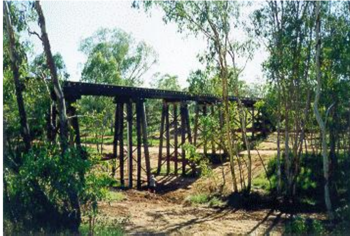
Plate 2 – ‘Alpha’ River Height Flood Warning Station (Photograph courtesy of Bureau of Meteorology)
