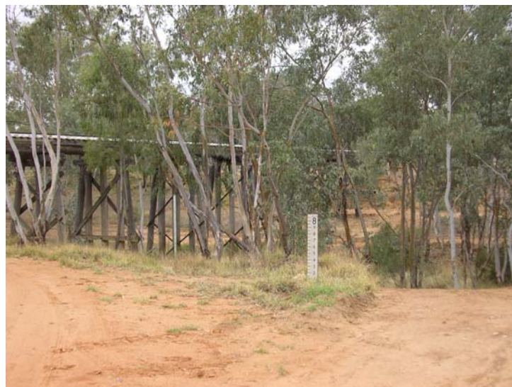
Plate 3 – ‘Alpha’ River Height Flood Warning Station
