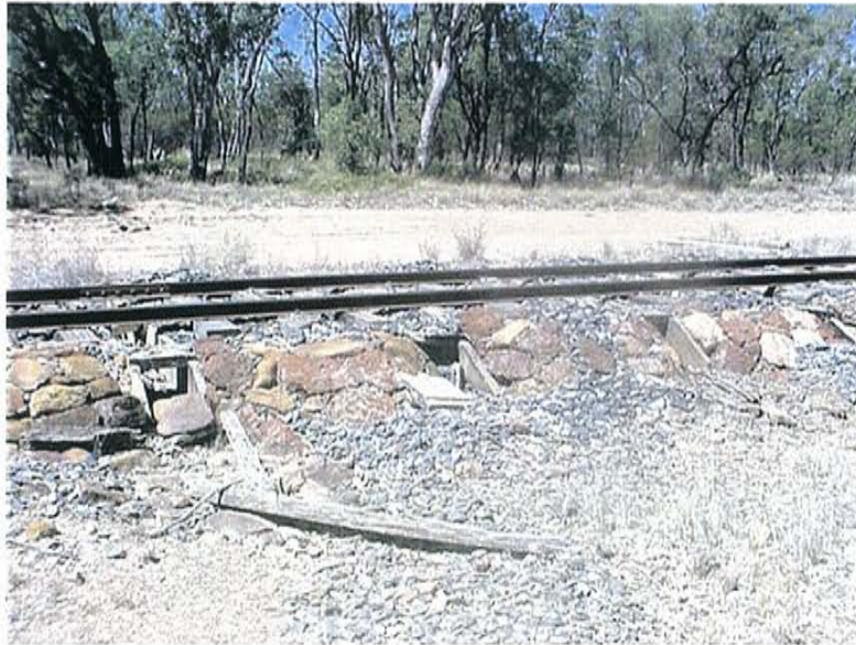
Plate 5 – Culverts (Shutes) under railway
