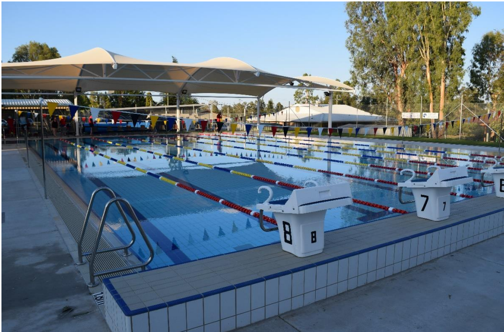
Alpha Memorial Pool - completed October 2015
