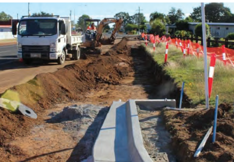
Above: Capital works in Box Street, Barcaldine.
