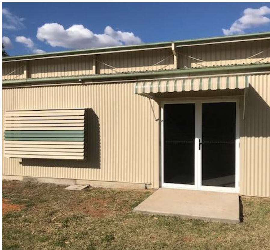
The Alpha Showground Grandstand and Kitchen awning.
