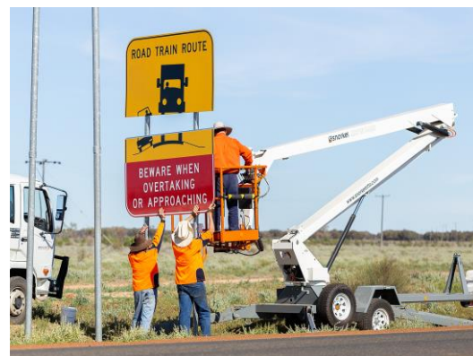
Sign replacement on Barcaldine-Aramac Road.
