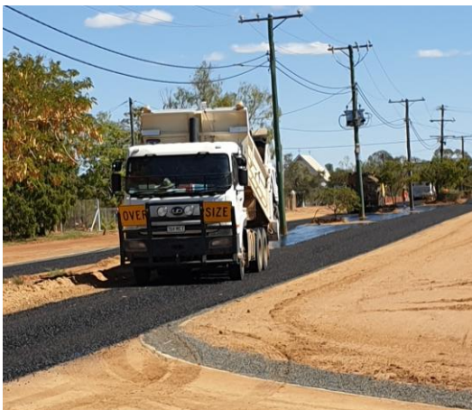
Roadworks in Sword Street, Muttaborra.
