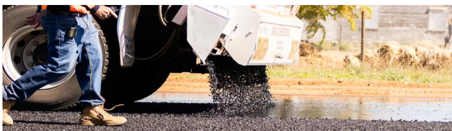
Roadworks in Porter Street, Aramac.
