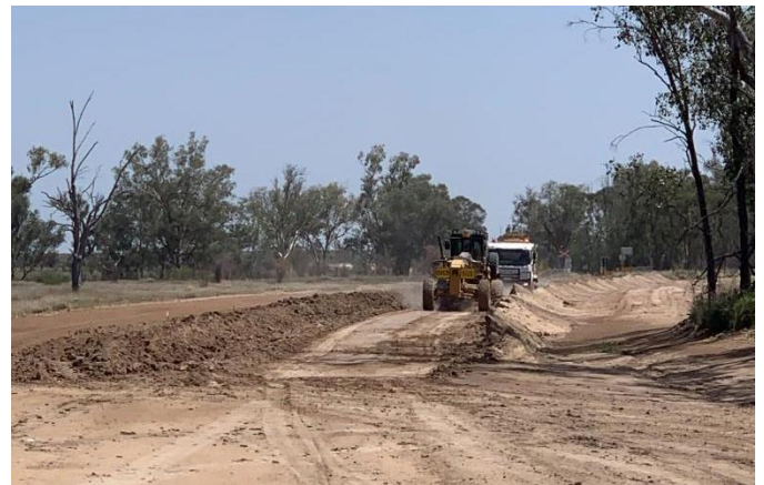
Pine Hill Roadworks, Alpha.
