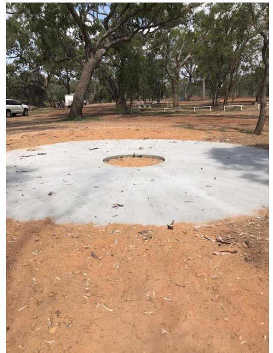
New fire pit construction at Redbank Park, Jericho.
